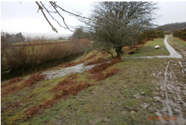
Plate 10/P3: View north along western side of tramway showing surface water run-off flowing down the tramway ruts from north of the existing quarry then flowing downslope towards the Leat.
