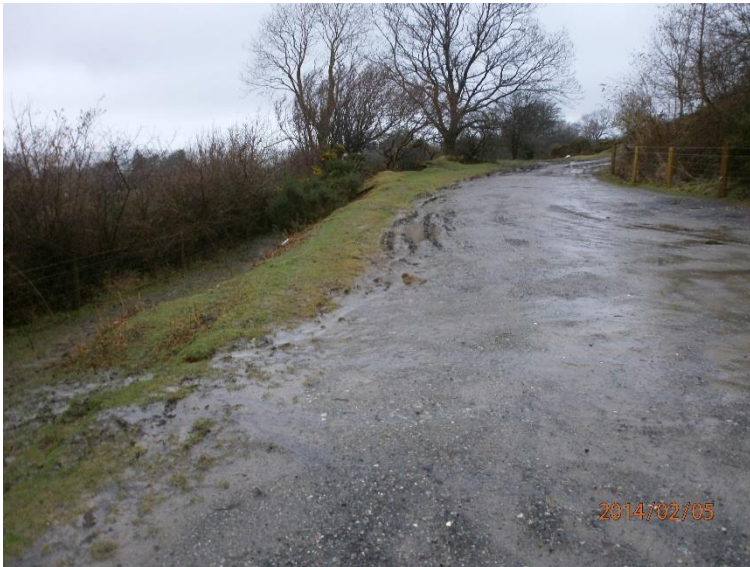
Plate 10/P5: Access road adjacent to quarry entrance showing no significant surface water run-off.
